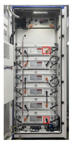
Figure 59: Battery Cluster Positive and Negative Plugs Locations
