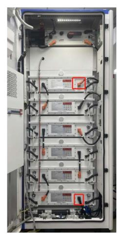
Figure 64: Battery Cluster Positive and Negative Bus Plug Locations
