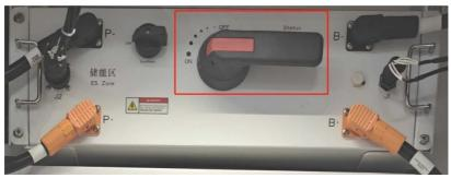
Figure 61: Battery Disconnect Switch QB in High Voltage Box
