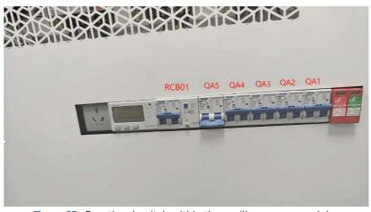
Figure 65: Functional switch within the auxiliary power module
