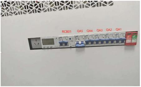
Figure 60: Switches in the auxiliary power module
