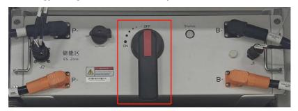
Figure 63: High Voltage Box Battery Disconnect Switch QB
